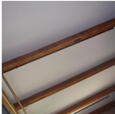
4. Fire Sprinkler - Reinstalled
