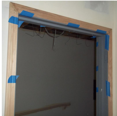
5. Wood Casing Install
