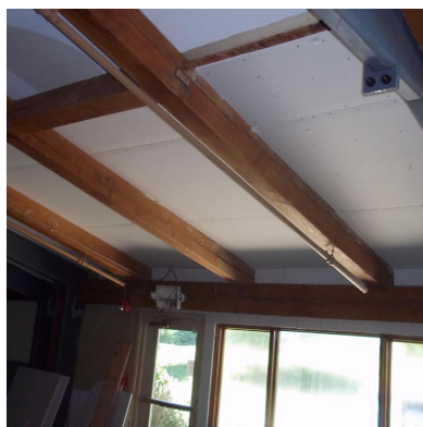
3. Drywall Install Board Room
